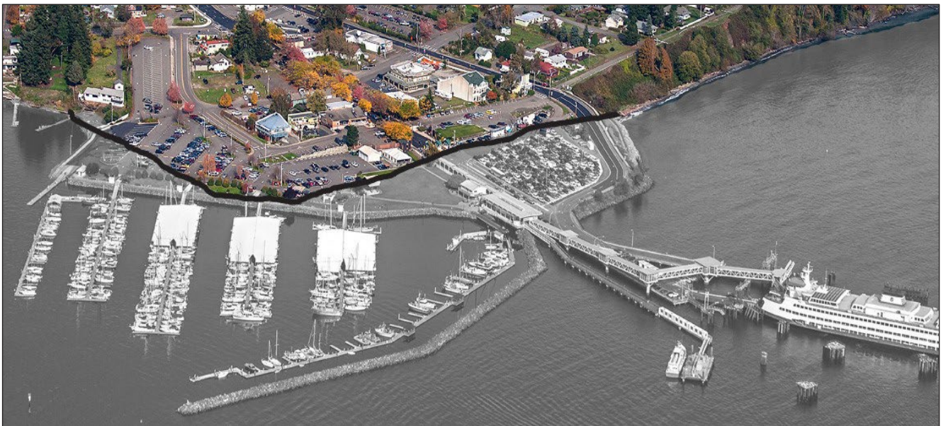
The original Kingston shoreline prior to 1965 when the U.S. Army Corps of Engineers built the breakwater, dredged the harbor area, and used the fill to construct what is now the marina, Mike Wallace Park and the WSDOT ferry terminal and parking lot.
