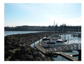
**Breakwater and Harbor** Construction began in 1966 with the breakwater and ended in 1967 with completion of harbor dredging. The purpose of the breakwater is to allow protection for marina facilities from waves of storms and ships, to slow the accumulation of sediment by slowing water flow rates with tides, and to protect boats from material drift. Total length of the breakwater is 1,040 feet.
