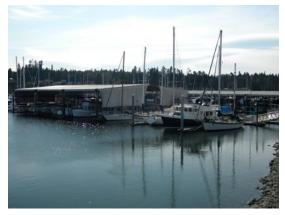
**Permanent Moorage** consists of five floating piers. The main piers are lettered A through E from west to east and the slips of each pier increase in size to the east. Total permanent moorage is currently 261 slips. The original permanent moorage floats were built of wood in 1967. In 1985 the floats were upgraded to concrete. Fresh water runs down one side of each dock. Electrical pedestals with meters supply 30 amps of power for each slip.
